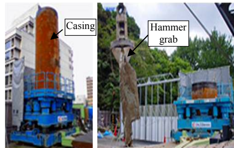
Figure 14. Rotary all casing boring machine.
