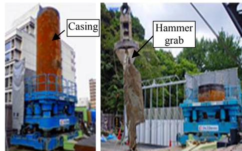
Figure 14. Rotary all casing boring machine.
